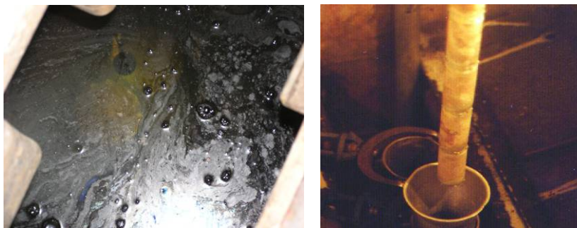
Fig. 4. Cooling pool water and damaged SFAs.
