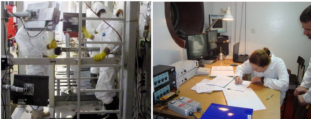
Fig. 7. Working frame tower and operator's room
