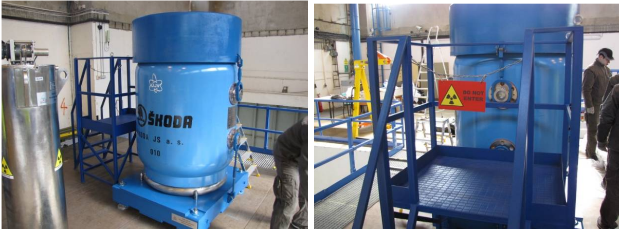
Fig. 4. Equipment installation at UJV
