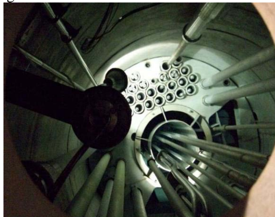
b – reactor pool
