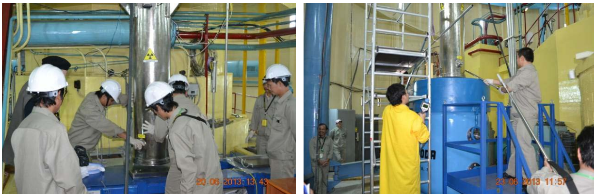
Fig. 6. Practicing in loading VVR-M2 SFAs into the shipping cask
