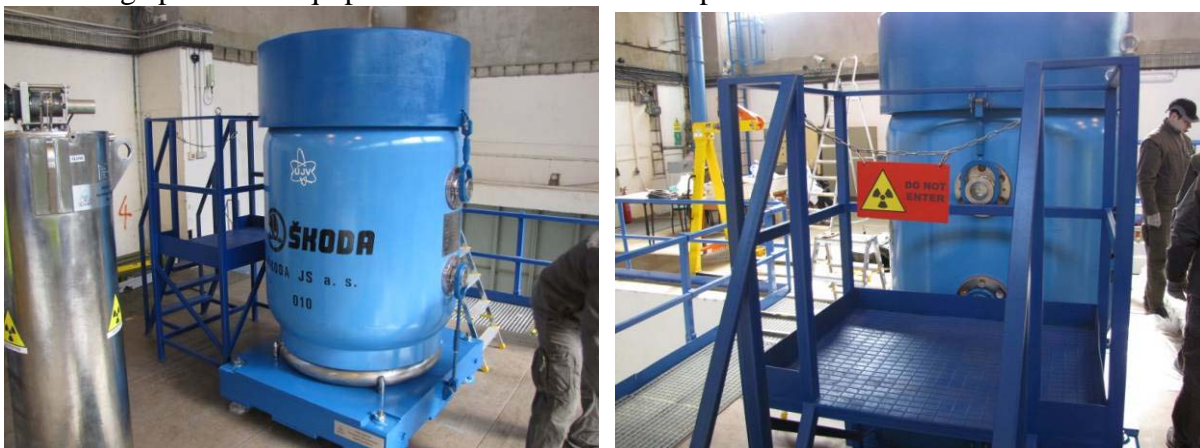
Fig. 4. Equipment installation at UJV
