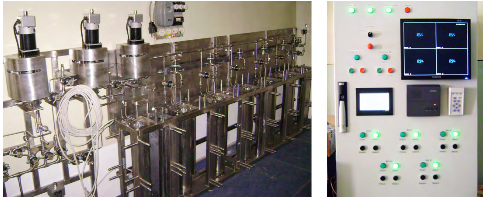
Figure 1 Partly-mounted equipment for liquid spent fuel discharge and temporary storage in the reactor hall
