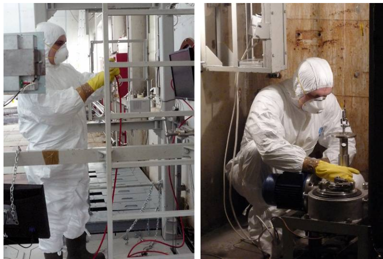
Fig.4. Mounting the equipment
