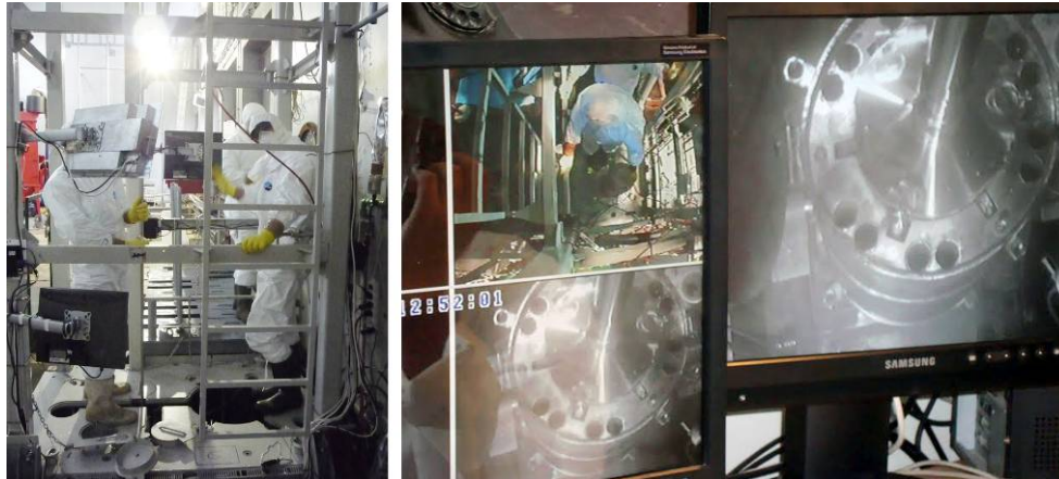
Fig.5. SNF repackaging operations on the working frame
