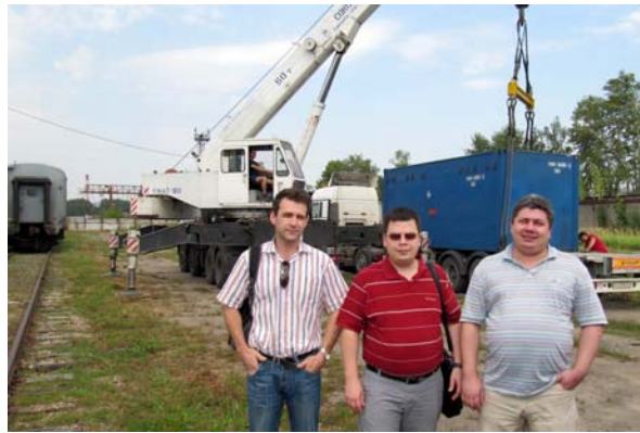
Fig.9. Reloading the containers with SNF from trucks onto rail flatcars
