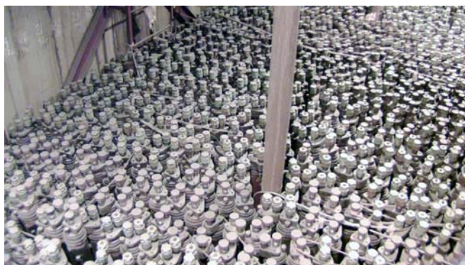
Fig. 1. Layout of SFAs in the drained storage pool
