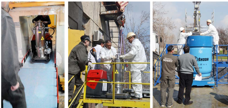
Fig.8. Dry Runs of equipment on site of IIN-3M reactor
