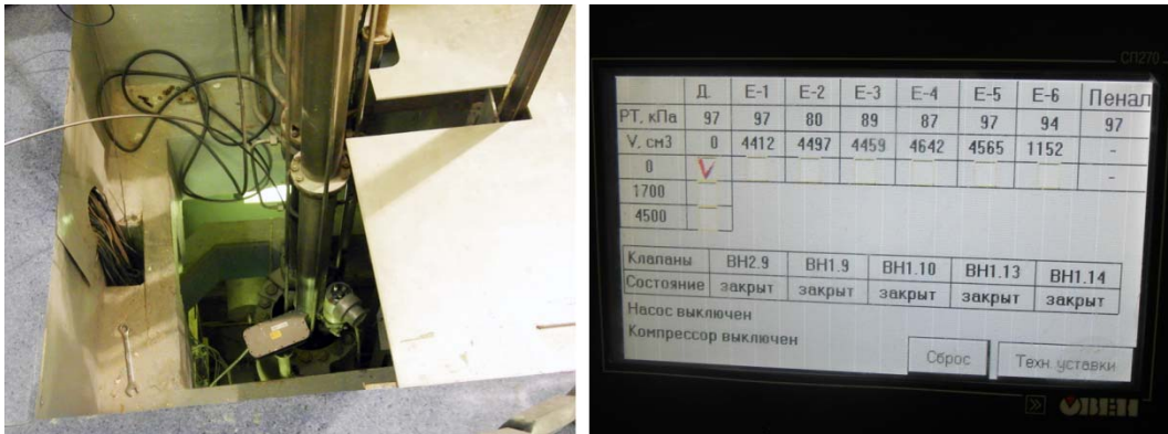
Fig. 2. IIN-3M reactor. Readings on the control monitor during the LSNF discharge from the reactor
