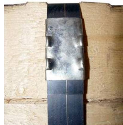
Fig. 6. Brace used for fixing the clamp ends
